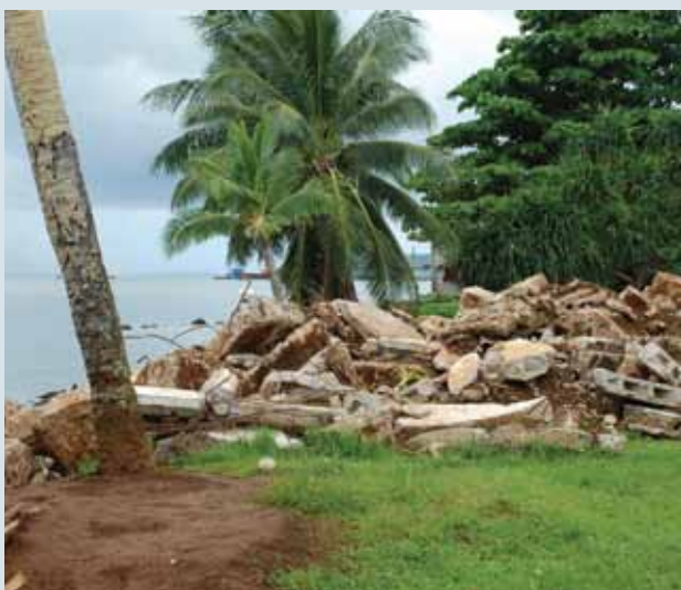
Shoring using building debris (Liku)
