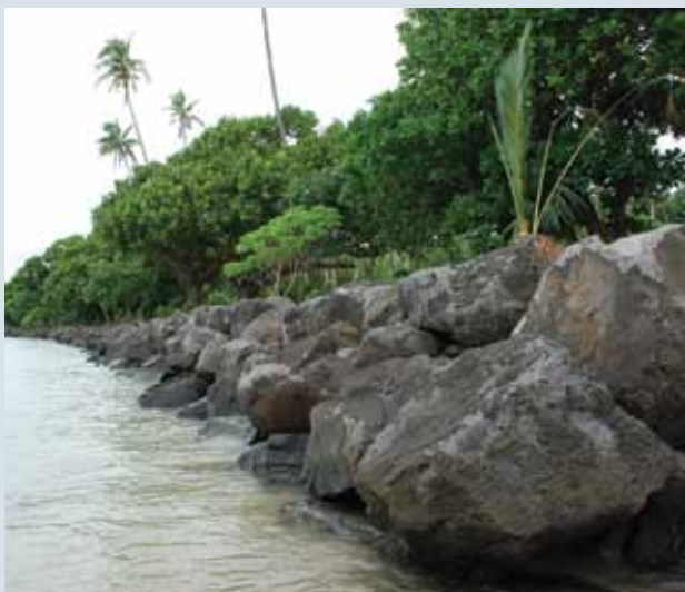
Shoring up the sea front (Vaitapu)
